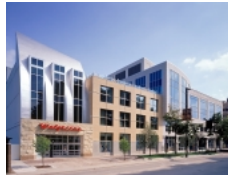
This Walgreen's on Main St. facing the Capitol is fronted with a curved aluminum facade over a cut-stone base.
